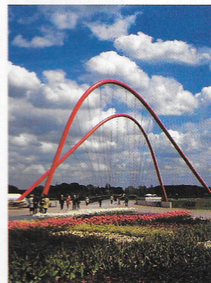
New pedestrian connections (top) and engineering structures (above)
